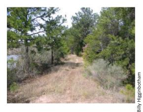
This fish pond dam likely will have problems with leakage (if not already) and breakage if the trees are not killed or removed.
