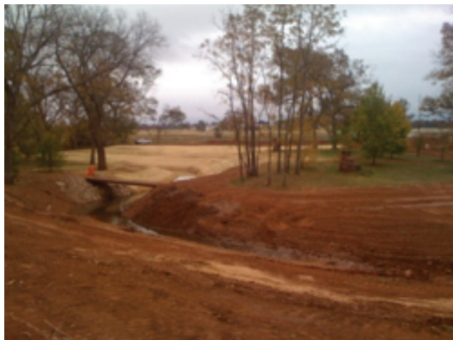
Figure 6. A bank that has been re-sloped. Vegetation will be added once construction is complete.
