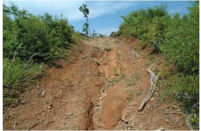
*Forest roads should not be constructed perpendicular to slope. Roads such as this should be closed and planted to trees or shrubs.*
